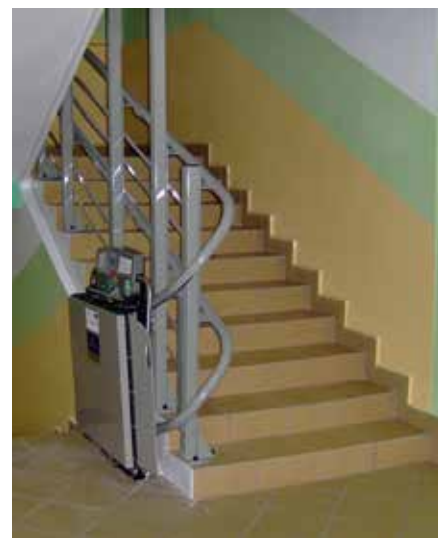
Fixing into the stairwell
