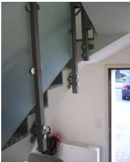
Fixing on stair stringer
