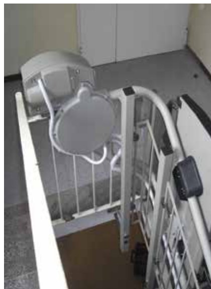
90° drive in the eye of the stair.
