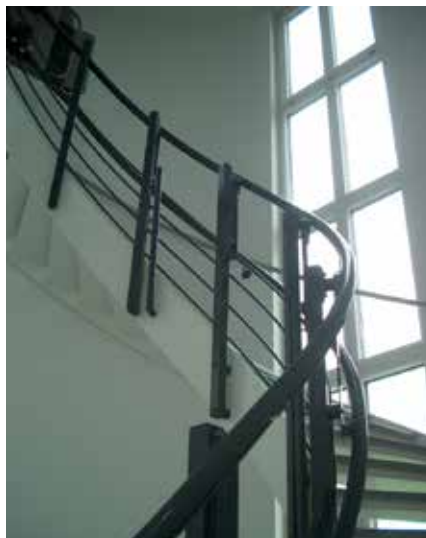
Fixing on the stringer
